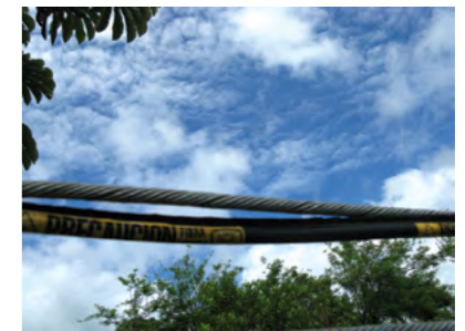
■ ICE-Figure-8 Self-supporting Cable
