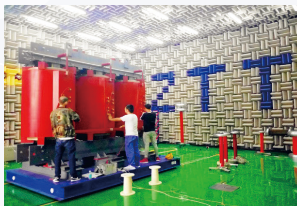
Noise test hall
