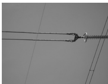
Dead-end for ACSR conductor
