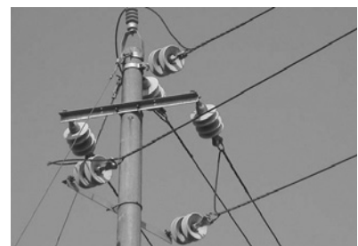
Dead-end for AAC conductor
